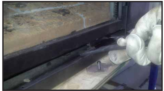
Figure 14.7. Glass Clip Tool Location
